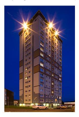
As well as the five colours used in Motherwell, Steni's lightweight Nature panels are available in another 19 colours and five grades of stone sourced from varying areas of Europe. The panels are Class O fire resistant as well as resistant to weather, rot and aggressive environments.
