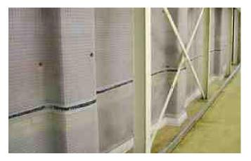
Stonehouse Basements was able to offer a quick and clean waterproofing solution without extensive preparation works as would have been the case with a tanking alternative.
