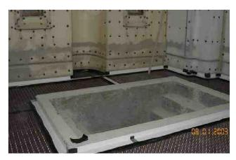
The floor areas were protected with Newton 520 as a lost drainage layer as the integrity of the RC slab was in question. Insulation was then deployed on the 520 with Newton 501 Slimline installed above as an effective dpm. A 65mm screed and floating floor was then chosen as the final floor finish to the project. A
