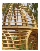
All joints of the arched timbers are scarfed to create the tight curve and pegged using the traditional framing pegs.
