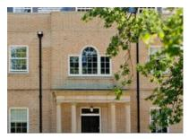
Additional fenestration also specified was a bespoke fixed casement ornamental arched window. Positioned central to the frontage, this window floods the upper landing with natural light. A Westbury Oak conservation entrance door, finished in black stain, provides a fitting grand aesthetic to the property's frontage.
