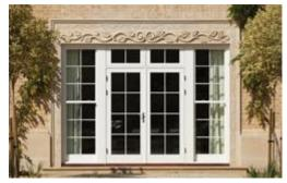
Made using engineered timber for its durability and stability, the windows feature traditional 'weights and cords' mechanism and polished chrome ironmongery. The window design was carried throughout to include full height sash windows as sidelights beside the French doors to the rear ground floor.
