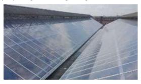
The 10,500 m2 single-layer Texlon<sup>®</sup> EFTE foil system installed at Carlisle Citadel Station is formed of 10 metre by 5 metre extruded ETFE sheets. Each has a thickness of just 250 microns. Each ETFE sheet is welded along its perimeter to form an edge that can be folded over a 'Keder' extrusion rod. The perimeter assembly enables a structural connection between the ETFE panel and the aluminium perimeter framing.
