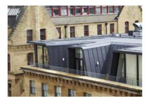
Kraus Schönberg Architects' sophisticated design for the Garbe Group involved complete refurbishment and the addition of a roof extension. However, because of the building's listing, the  $1300 \mathrm{m}^2$  zinc and engineered timber roof was designed to be self-supporting. A further requirement of the conversion to high specification apartments was to use a sustainable, high performance material with proven colour retention.
