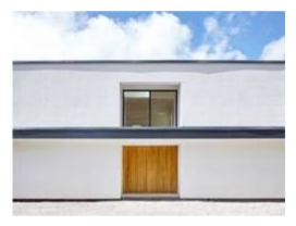
To achieve the minimal design, the door is flush to the frame, and to the adjacent cladding which fundamentally hides an internal room but also enlarges the front entrance. To further increase the minimal feel of the entrance, Urban Front's Option 20 handle, the concealed handle, was specified and also adds to the beauty of the finished doorset.
