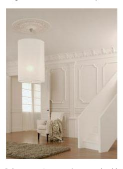
Polymer cornices are also more durable than plaster and, not being brittle, are less prone to damage. They are pre-primed to require just one coat of paint, unlike plaster that can soak up several coats. The cornices are installed simply by using adhesives, and any gaps or joints can be quickly and easily filled for a perfect finish.
