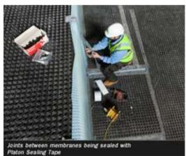
The Type C system comprised BBA certified Platon P8 cavity drain membrane to the floor and BBA certified Platon P20 cavity drain membrane to the walls. Perimeter channels were formed to house Triton Aqua Channel drainage conduit to divert any water entering behind or beneath the membranes to the sump and pump system. To allow for maintenance of the system, rodding eyes were installed to the Aqua Channel every 10 linear metres.
