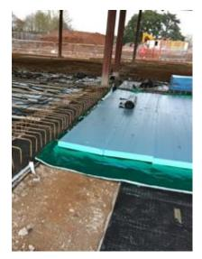
The system comprised Triton's <u>TGS-GV25</u>, a 25mm thick, single sided geo-composite that provides a void beneath the floor slab and, when connected to the air venting system, allows sufficient air changes to dilute any gases present. The TGS-GV25 was installed in strips at 6 metre centres across the site and linked to ground level vent boxes before the installation of insulation and <u>Triton's TGS-HP750 membrane</u> as a gas and waterproofing barrier.
