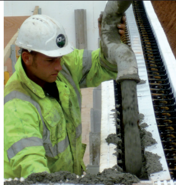
Triton's watertight concrete system conforms to Type B waterproofing as defined by BS 8102 2009
