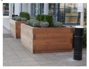
Townscape designed a hardwood FSC certified sapele timber surround to encase the CT Block system to create a planter, complete with a planting membrane and drainage material. The CT Block itself required only the usual 100mm recession, meaning installation was quick and cost effective.
