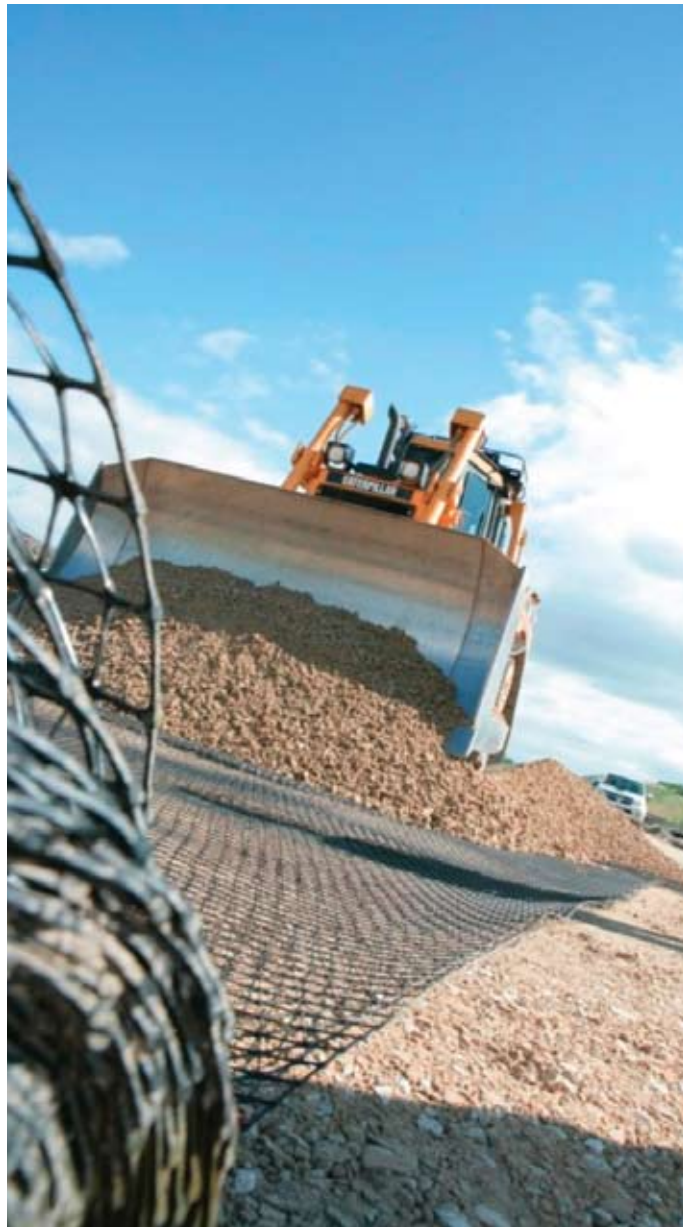
For a new link road built by Costain over marshland near Wakefield, the performance of Tensar TriAx™ demonstrated clear performance advantages
