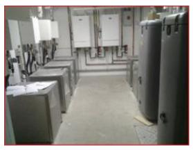
The care home is also equipped with two Keston Gas boilers (installed by a separate company) as a back up system.
