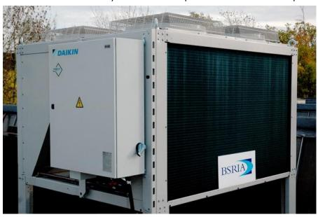
As BSRIA also had an occasional requirement for low water temperature operation, Space Air recommended a Daikin EWAQ100 DAYNP with 'ZL' control software to allow the set point to be reduced when required. This optimised R410A chiller features a dual brazed plate heat exchanger and was supplied with fully integrated hydronics. It offers an ESEER of 3.8 even at minus 5°degrees C LWT and was delivered and commissioned by Space Air within 5 weeks of the original enquiry.
