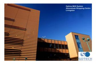
As well as being the more cost-effective, Sotech's Optima Baguette Sunscreen is also fully-recyclable and can, with a module measuring 2.7m by 1.8m weighing just 40kg, be factory-assembled for faster fitting on site.
