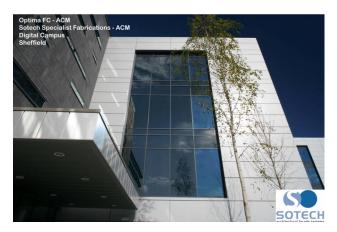
Specified in a modern anodic silver finish designed to replicate a stainless steel appearance and measuring up to 5.5m in length, the large flat panels have been used to create a striking 'wrap around' cladding effect that provides seamless integration between the different elevations. Sotech also designed and manufactured PPC feature flashings to complete the look.
