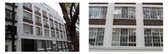
Evolution takes inspiration from traditional steel windows offering signature slim profiles that maximise glazing sightlines coupled with advanced aluminium polyamide thermal break technology. These credentials make Evolution the perfect choice for heritage applications where the refurbishment of traditional steel windows requires a prestigious system with the performance of modern thermally broken aluminium.
