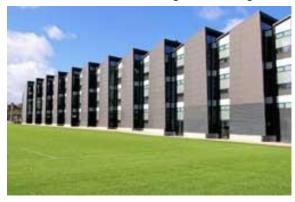
west elevations there are external solar fins (or shades) to protect against excessive glare and heat gain; and the curtain walling specification incorporates opaque insulated glazed units which minimise excessive heat loss in winter. Internal ducts enable the deep plan workshops to be naturally ventilated, reducing the requirement for mechanical ventilation.
