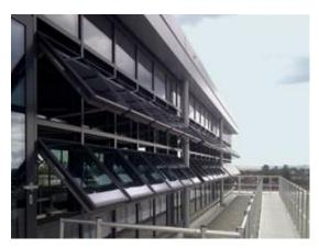
Four separate atrium spaces feature as part of the building, designed by AWW Architects, and each incorporates 84 Schüco AWS 102 projected top hung vents. The vents are automatically operated by a total of 336 SCCO 24 30 concealed actuators, which were supplied, installed and commissioned by SE Controls in partnership with specialist façade contractor, Norking Aluminium.
