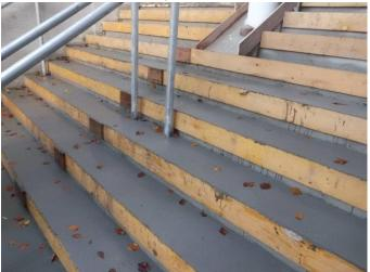
the venue, to provide a hard wearing, dust proof, waterproof surface that could be laid in thin section. The screed was installed by sub contractor Industrial Floor Treatments.
