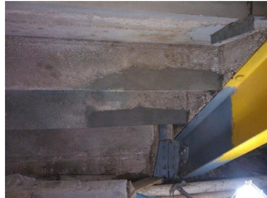
The same area after application of the repair mortar
