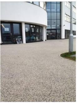
RonaDeck Resin Bound Surfacing is a hard wearing, SuDS compliant alternative to traditional paving and has the attractiveness of natural aggregate while being easily maintained unlike loose gravel. It is also suitable for wheel chairs and is slip-resistant.
