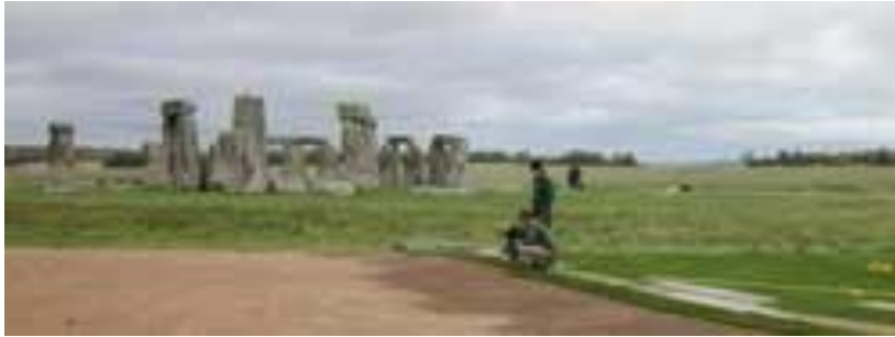
Parsons Landscapes staff laying Rolawn turf at Stonehenge
