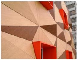
Several triangles were cut from each façade board, each one slightly different across the whole façade. Despite being lightweight, ROCKPANEL is as robust as stone. Its weather and moisture resistant properties ensure that the edges of the boards do not need to be treated – saving time and cost.
