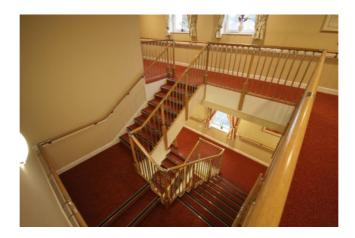
FUSION® Commercial stair balustrade was installed on the main staircase to provide a safe and stylish barrier. The system's combination of minimalist oak handrails and sleek tubular balusters in a contemporary brushed nickel finish complemented the building's modern décor and other good quality furnishings, whilst its availability off-the-shelf meant there were no lengthy lead times.
