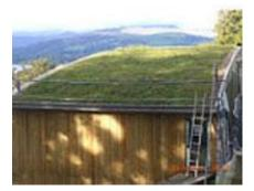
In order to blend into the hillside setting, the domed roofs of the house were to be covered with a wildflower meadow mix to provide a green roof construction. The Protec System was chosen as a waterproofing membrane for the roofs as it is ideally suited for green roof applications. Lightweight, flexible and highly durable, the system can easily accommodate structural expansion movements and is tough enough to resist root penetration.
