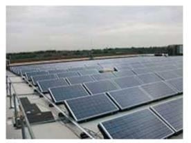
288 PV solar panels were then installed over the Protec membrane which are set to generate 62,000 kWh per year, which equates to around  $\pounds$ 23,000 -  $\pounds$ 25,000 of annual savings for Eastleigh Borough Council. What's more, the expected payback of the panels is a mere 8 or 9 years.
