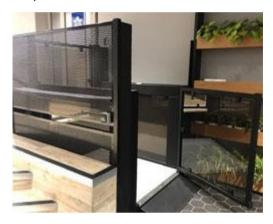
Platform Lift Company designed and built a bespoke platform lift solution. To create an open and modern feel to the lift, glass was used for the door and car, and steel black mesh for the sides. Installation was carried out over two days.
