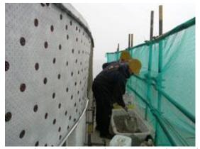
render finish. Mechanically fixed at 100mm - 150mm centres, the meshed membrane was applied and a 6:1:1 clean sharp sand, cement, lime mix was then applied in two 6mm coats. A rubbed float finish was then applied prior to decoration with a high build flexible and breathable masonry paint.
