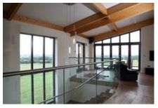
Mumford & Wood's double glazed Contemporary<sup>TM</sup> windows and doors are BSI 'A – C' energy rated, depending on specification, and achieves an overall frame U-value of 1.4 W/m<sup>2</sup>.K. This satisfies current Part L Building Regulations 2010 and surpasses the requirements of the forthcoming 2013 Regulations.
