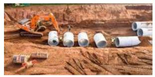
Severn Trent Water contracted NMC Nomenca to deliver a solution that saw the installation of fifty 1500mm and ninety-nine 1800mm precast concrete pipes, some of which were laid as a multi-tank system to improve the management of water ensuring that the day-to-day life of the community is not disturbed by flooding.
