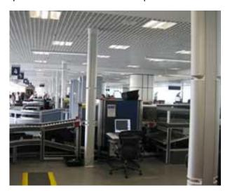
Birmingham Airport's Terminal electrical engineer Mohammed Benyahia, said: "The use of Powerpoles provides the correct solution for the provision of power and data to the security equipment, whilst also keeping cable lengths to a minimum and eliminating trip hazards in this very busy area of the airport. We are very pleased with the end result."
