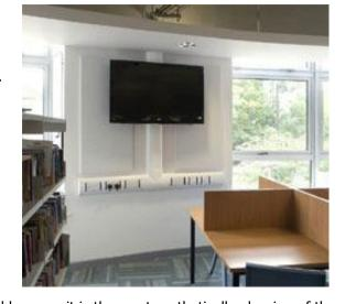
because it is CAT 6 compliant, easy to install and because it is the most aesthetically pleasing of the containment systems we have looked at - and we have looked at quite a few! The client is happy with it and we are happy with it. As a result of the effectiveness of both systems, we are taking them through other schools within the BSF initiative."
