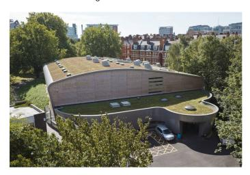
Explaining the reasoning behind the use of natural daylight, Mark Hewitt of LCE says the Monodraught Sunpipes diffuse daylight, avoiding problems such as glare and contrast that are often experienced with direct sunlight from windows, and which can interfere with sporting activities.
