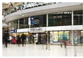
This was especially significant on the concourse level retail units where toughened, heat soak tested, and laminated structural glass was installed with associated support fins, brackets, perimeter channels, and metal louvres. The 21.5mm thick glass was carefully calculated to sustain the required structural loads, and in places reached up to 5 metres high. Around the three ATM locations, there is
