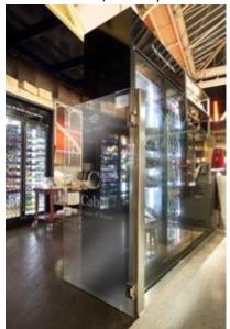
also featured back painted, toughened glass wall cladding. The use of structural glass continued to the mezzanine level retail units where a combination of toughened and laminated glass assemblies form the shop fronts and feature in the frameless glass doors.
