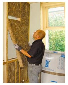
benefited from insulation as well as a seal around the hatch, eliminating any cold areas and draughts. Knauf Insulation's Loft Roll 44 is a low density glass mineral wool roll, which is lightweight, flexible, resilient and non-combustible.
