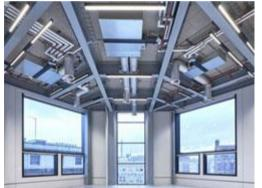
One major challenge was to find a material for the ceilings that would complement the exposed services and an industrial design aesthetic, whilst fulfilling modern acoustic requirements. Heradesign with its outstanding acoustic credentials and raw wood wool texture ticked all the boxes. Specified in Grey, Heradesign provided a strong visual contrast to the exposed structural elements. 4000m2 Knauf AMF Heradesign was employed.
