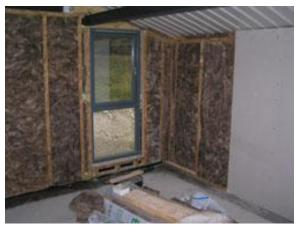
With walls only built to one metre tall and the upper part of the barn constructed from a steel frame, the structure would have to be filled in to full height before it could be insulated.
