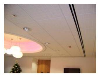
Available as both tiles and planks, in a range of edge details and module sizes, Thermatex Symetra offers architects and designers even greater flexibility and scope for contemporary ceiling design. Performance is not compromised as the Thermatex Symetra range provides high levels of sound absorption, good fire protection and excellent light reflection.
