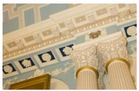
These were painted using a specialist 'wiped' technique to give a two-tone effect. At ground level the wooden wall panels had to be stripped back and re-varnished. In some areas, detailing was painted in gold.
