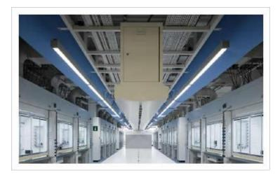
Other advantages of textile over metal include typically 50% savings on installation costs; higher duct velocities possible for low NR rated areas; ductwork requiring no insulation and supplied pre-finished in a range of colours; and very hygienic through ease of washing and maintenance. KE Fibertec designs and builds bespoke systems focused entirely on customer requirements. Installation is fast and simple, requiring no special tools.
