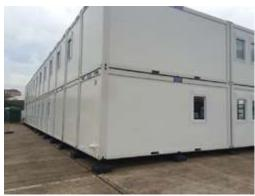
The double storey buildings by T F Jacksons provide all the space capacity required and if they need to be moved, the Jackpad system can be lifted with no damage to the substrate.
