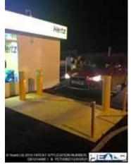
bollards remain visible to the user at all times, unlike traditional automated rising bollards. Achieving zero penetration and zero dispersion during PAS68 testing, the Matador presents a truly formidable defence against hostile vehicle attack.
