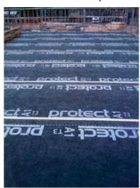
UV and heat stable, and completely waterproof, Protect A1 T3 can be used as a temporary roof covering for up to three months before the tiles or slates are laid. Once the roof is complete, Protect A1 T3 does not generate noise under wind gusting, and is certified for unrestricted use for wind uplift. Further, its absorbent undersurface prevents condensate drip-off, helping eliminate risk of damp issues in the roof, assuming appropriate high and low level roofspace ventilation is provided.
