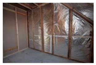
Each of the timber frame properties features Glidevale's innovative Protect TF200 Thermo reflective breather membrane and VC Foil low emissivity vapour control layer in the roofs and walls. The combination ensures optimum warmth is retained within the structure, air leakage is minimised, yet internal moisture vapour is ventilated out to atmosphere, minimising the risk of potential damp and condensation.
