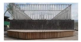
Measuring 35m in length, the bridge includes ornate laser cut steel panels and coloured resin strips within the balustrade uprights, through which sunlight passes to create coloured shadows during the day and which is illuminated at night by lighting within the handrails. The provision of new seating was central to the footbridge scheme.
