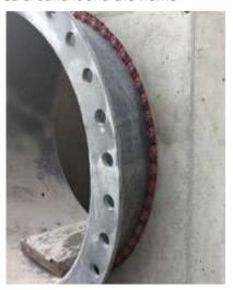
Flexseal provided the seal made to order, ensuring installation was as quick and efficient as possible. The contractors had no experience in fitting Ring Seals; however, installation was complete in less than 1 hour.
