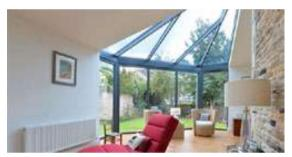
Rather than the extension containing a 90degree corner, it contains a glass hipped roof installed as a three section glass bay. Express bi-folding Doors manufactured and installed a steel portal frame for the roof to sit on. The body of the glass room contains three separate fixed picture windows creating a striking glass façade that looks great externally, whilst internally make the whole space feel larger, and much lighter.
